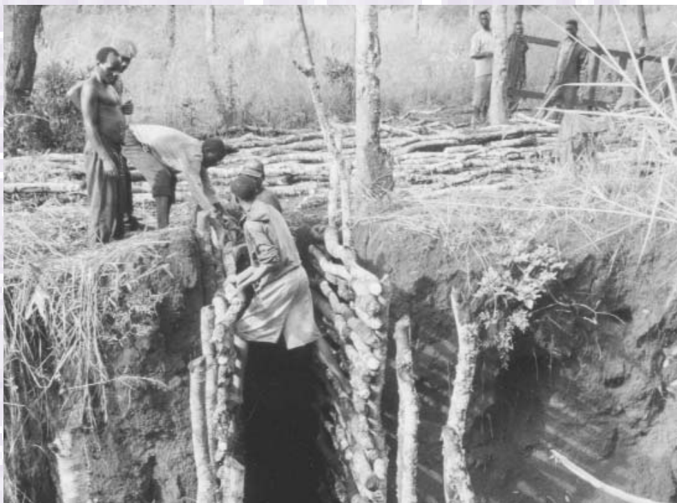
Poor site selection and planning can result in soil and gully erosion during heavy rains. Repairing the damage caused is expensive and time consuming.
